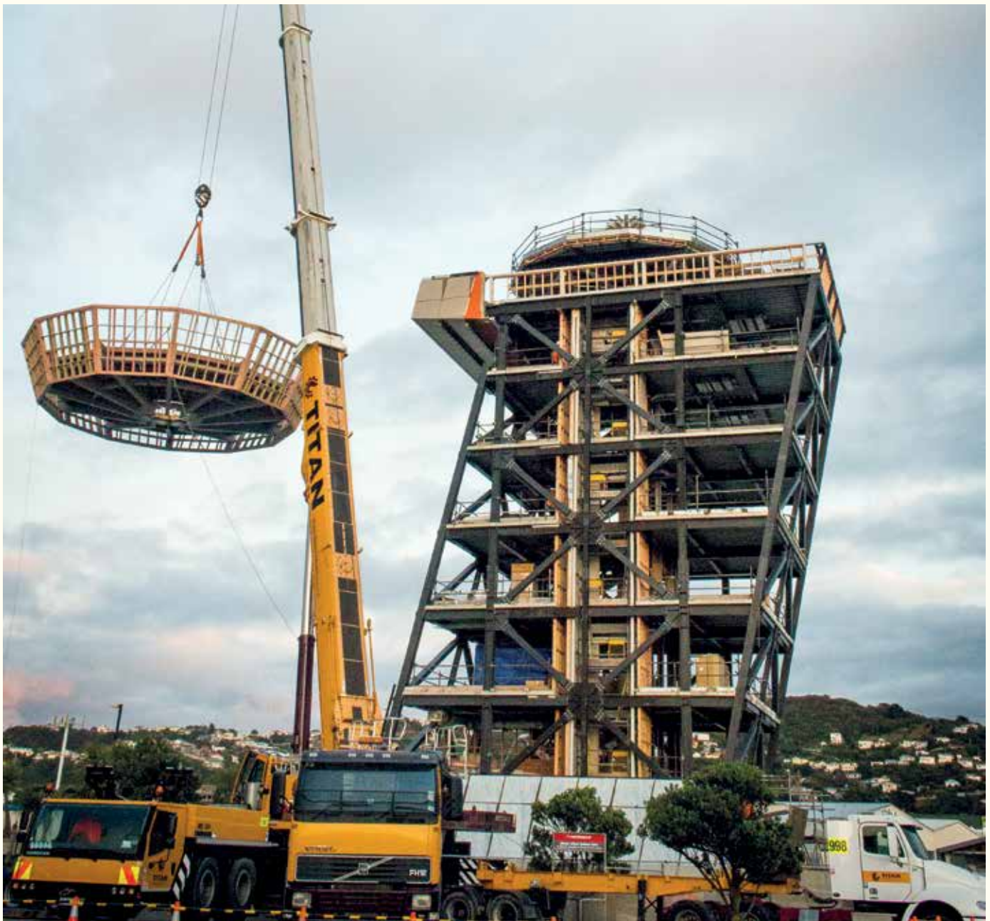
Wellington Tower build, May 2017
